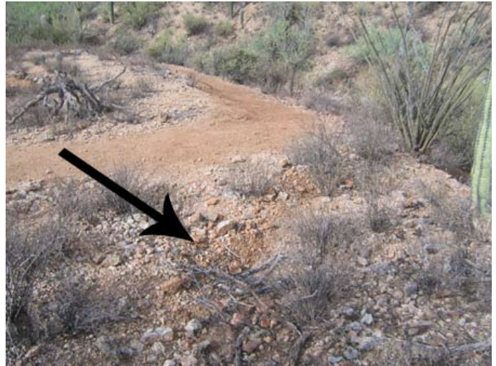
A few minutes with a McLeod was all it took to divert water off this embankment before it can get to the trail.
