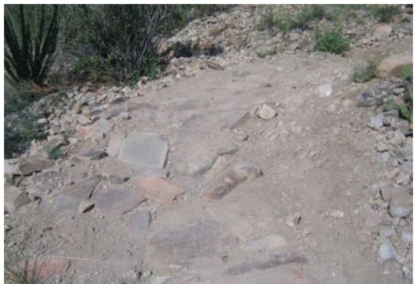
In places where the terrain forces the trail to run at a steep grade, an armored tread may provide a sustainable solution.
